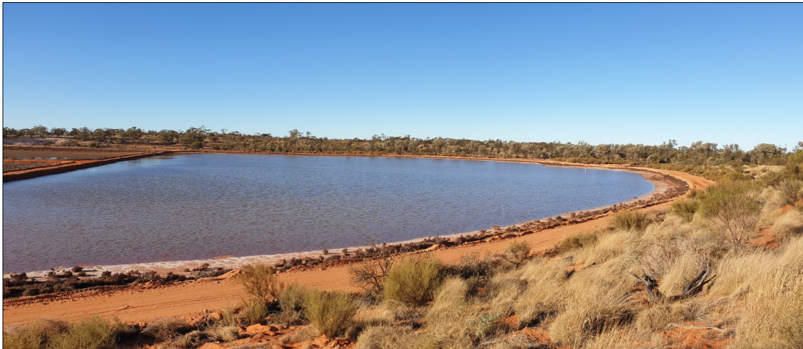
Figure 2: On-playa trial pre-concentration pond demonstrated low-cost, efficient lateral seepage barrier construction techniques, using the highly stable and easily accessible playa perimeter
