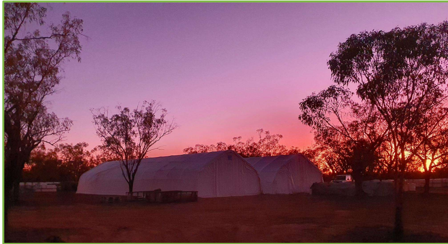
Figure 3: Construction of the new storage shelters at LSOP was completed during the period
