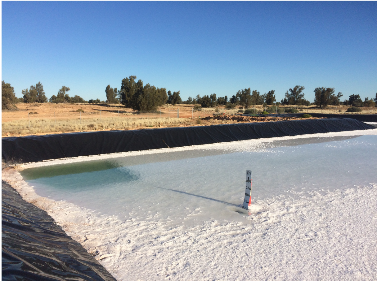
Figure 3: Pre-concentration pond after the transfer of concentrated brine to harvest pond 1, showing the crystallisation of 220 tonnes of predominantly sodium and magnesium salts on the base of the pond
