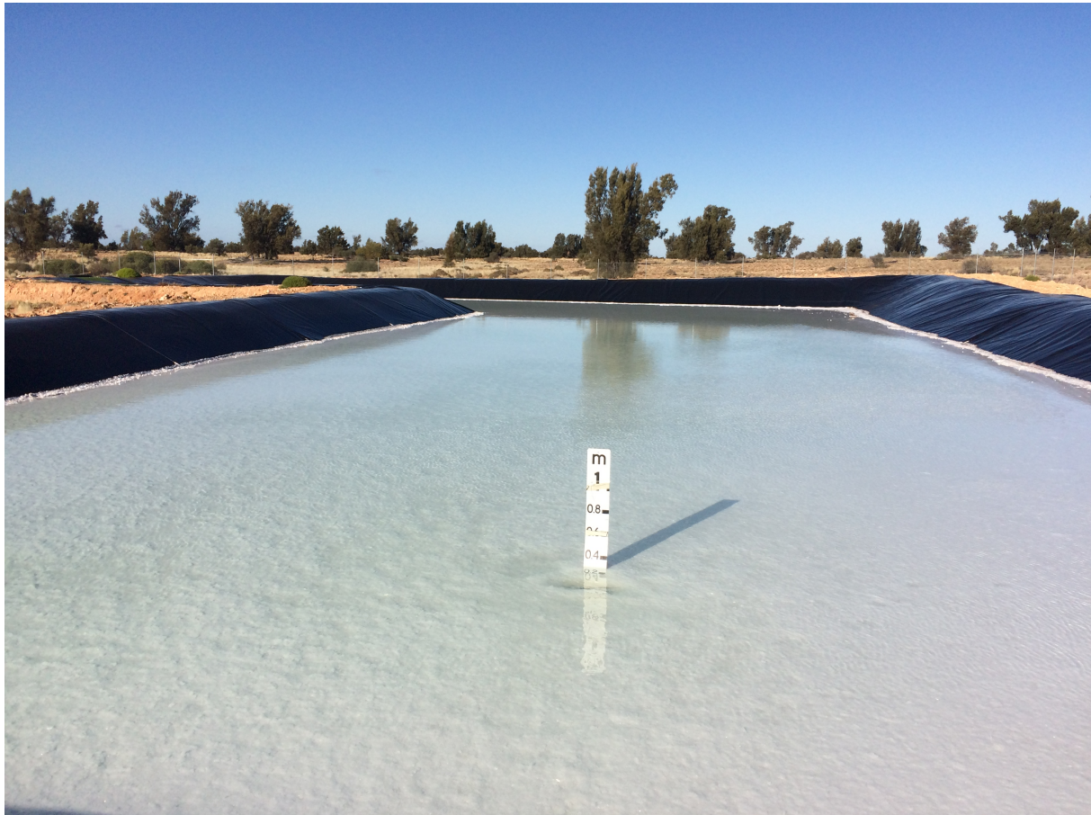
Figure 1: Pre-concentration pond at the Lake Wells SOP project prior to initial brine transfer
